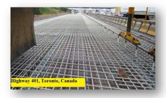
Composite reinforcement was used for construction of several pilot projects of Highway Bridges in Canada. Here, in the second part of 90's were put into commission 4 Highway Bridges with composite reinforcement applied during the construction (Manitoba Bridge, Saint-François Bridge, etc.).
